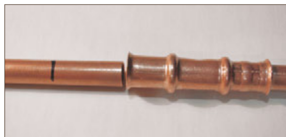
Figure 11.18. Tube marked for insertion into HVACR fitting
