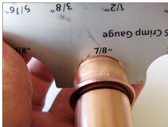
Figure 11.23. Correctly crimped fitting
