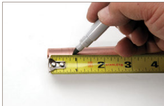
Figure 12.10. Making insertion depth
