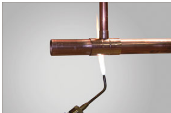
Figure 7.14. Preheating Fitting
