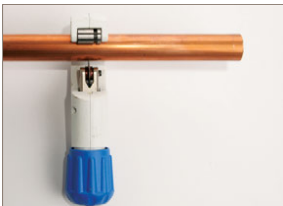
Figure 11.6. Cutting the tube square
