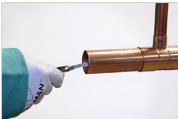
Figure 7.4. Reaming: Pocket Knife
