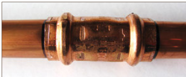
Figure 11.16. Completed installation of a press-connect joint
