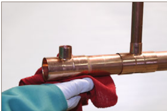
Figure 7.12. Removing Excess Flux
