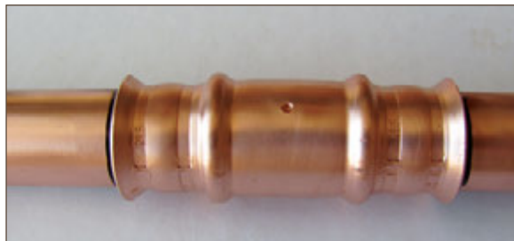
Figure 11.19. Completed joint with insertion marks visible
