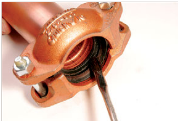
Figure 10.8. Applying lubrication to gasket
